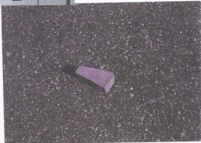
Concrete Sample on Asphalt Road Surface
