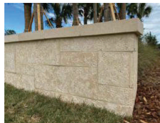
WALL VENEER 1/2" VENEER MORTAR
